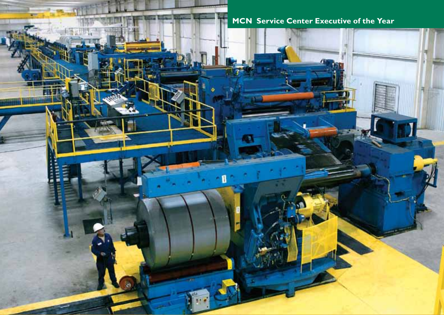
The pickling line at Heidtman's Cleveland plant was commissioned in 2005. It can handle coils up to 0.625-inch thick and 72 inches wide. It includes a Bradbury hydraulic leveler and a Parsytec continuous surface inspection system. (Photo courtesy Heidtman)
